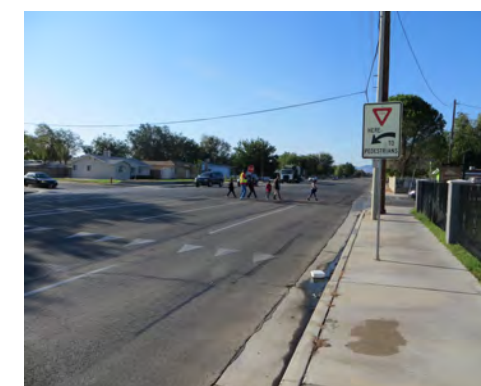
Advanced Stop Line
